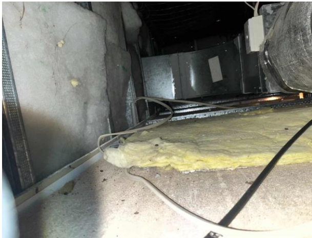
Line ID 68: Internal, Cancer Care Unit, East and West Sides, Throughout Ceiling Space, Insulation Batts - Suspected SMF
