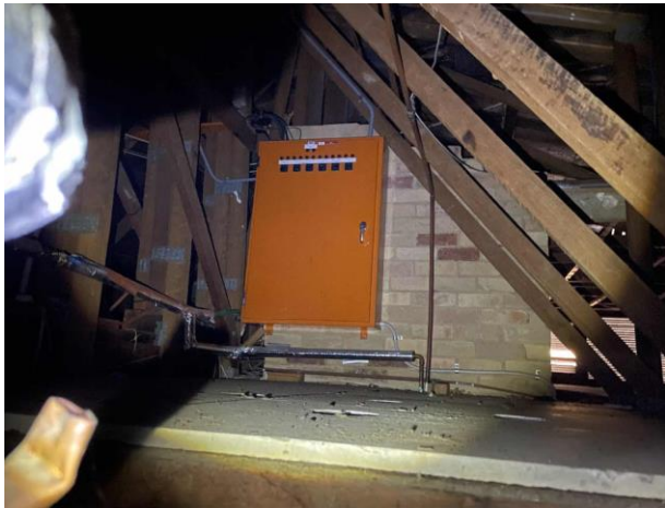
Line ID 38: Internal, Paediatric Unit, Ceiling Space, Switchboard, Bituminous Backing Board - Suspected Asbestos
