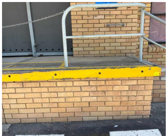
Line ID 52: External, Paediatric Unit, Eastern Side, to Timber, Yellow Paint - Lead Detected (1.8% w/w)
