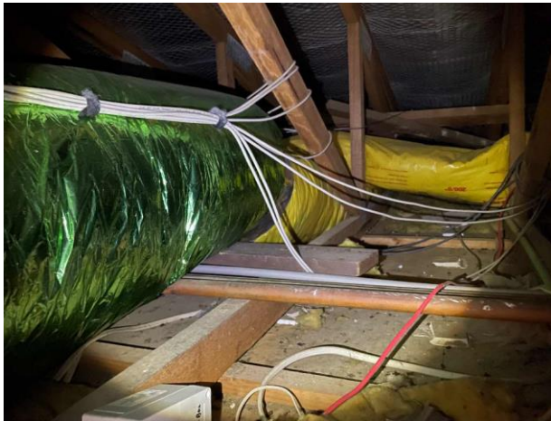
Line ID 80: Internal, Paediatric Unit, Ceiling Space, Flexible Ductwork Throughout, Insulation Material - Suspected SMF
