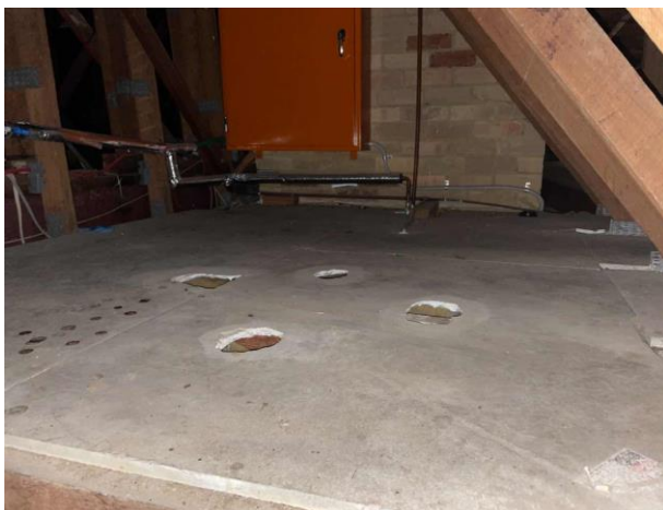
Line ID 36: Internal, Paediatric Unit, Ceiling Space, Central Area, Floor, Compressed Cement Sheet - Chrysotile Asbestos Detected
