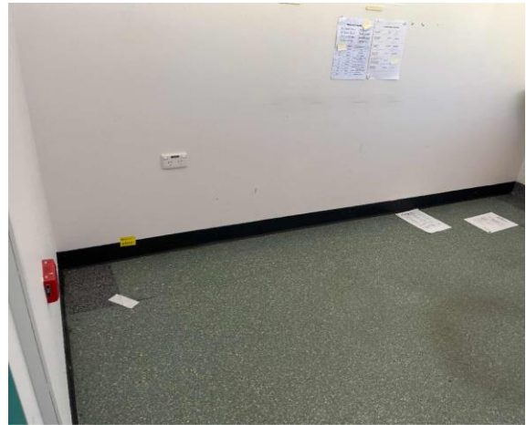
Line ID 42: Internal, Paediatric Unit, Room 8 30076, Below Green Vinyl, Paper Backing - Chrysotile Asbestos Detected
