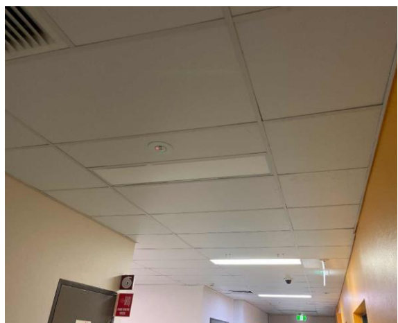
Line ID 79: Internal, Geriatric Unit Ground Level, Throughout, Hallways and Rooms, Compressed Ceiling Tiles - Suspected SMF
