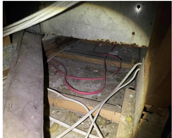
Line ID 40: Internal, Paediatric Unit, Central Corridor, Ceiling Space Above Plaster Ceiling, Below Compressed Panels, Fibre Cement Sheet - Chrysotile Asbestos Detected
