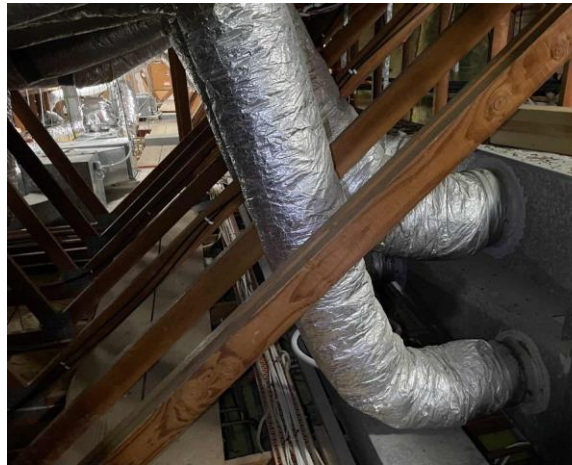
Line ID 71: Internal, Geriatric Unit, Rooftop Plant Rooms, Flexible Ductwork Throughout, Internal Insulation - Suspected SMF
