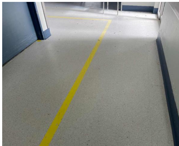
Line ID 29: Internal, Geriatric Unit Ground Level, Throughout, Floor Coverings, White Vinyl Sheet - No Asbestos Detected
