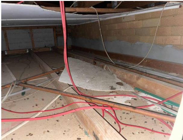
Line ID 32: Internal, Paediatric Unit, Adjacent NUM Room 30083, Ceiling Space, Fibre Cement Sheet Debris - Chrysotile Asbestos Detected
