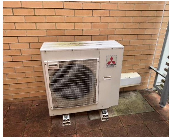
Line ID 87: External, Cancer Care Unit Ground Level, East Side, Mitsubishi AC Unit, R410A Hydrofluorocarbon (HFC) - Non ODS Refrigerant
