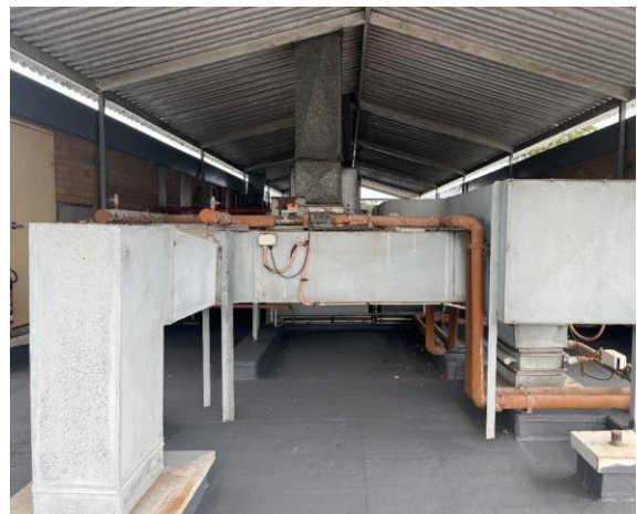
Line ID 60: External, Geriatric Unit Roof, Rooftop Plantroom, Ductwork Throughout, Internal Insulation - Suspected SMF
