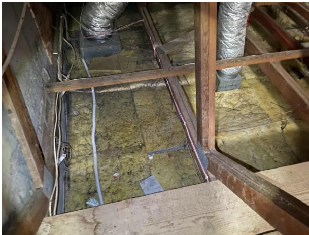
Line ID 74: Internal, Geriatric Unit, Rooftop Plant Rooms, Throughout Floor, Insulation Batts - Suspected SMF
