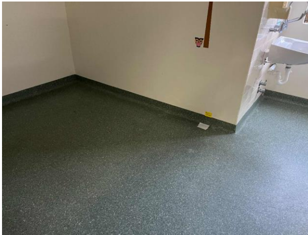
Line ID 47: Internal, Paediatric Unit, Throughout, Below Green Vinyl Sheet, Screed - Chrysotile Asbestos Detected
