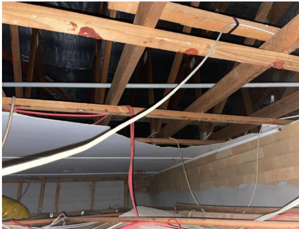
Line ID 33.1: Internal, Paediatric Unit, Adjacent NUM Room 30083, False Ceiling, Fibre Cement Sheet - Chrysotile Asbestos Detected
