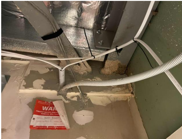
Line ID 26: Internal, Geriatric Unit Ground Level, Meeting Room, to Beams, Vermiculite - No Asbestos Detected
