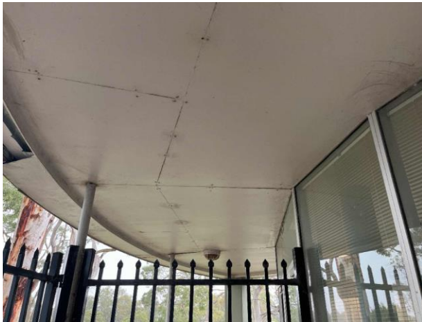
Line ID 3: External, Geriatric Unit Ground Level, Throughout, Awning, Fibre Cement Sheet - No Asbestos Detected
