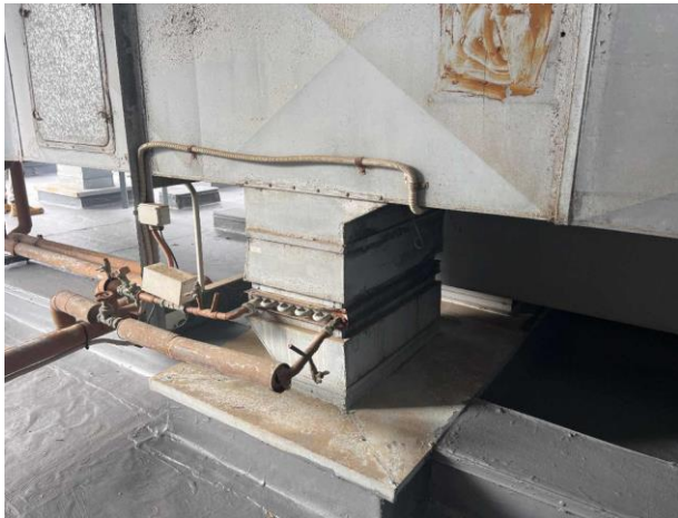
Line ID 7: External, Geriatric Unit Roof, Rooftop Plantroom, Within Eastern Ductwork, Millboard Insulation to Heating Coils - Suspected Asbestos
