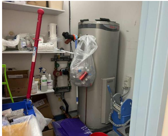
Line ID 62: Internal, Cancer Care Unit, Cleaners Room, Hot Water Heater, Internal Insulation - Suspected SMF
