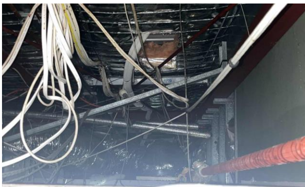
Line ID 63: Internal, Cancer Care Unit, East and West Sides, Ceiling, Compressed Ceiling Tiles - Suspected SMF
