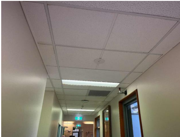
Line ID 63: Internal, Cancer Care Unit, East and West Sides, Ceiling, Compressed Ceiling Tiles - Suspected SMF
