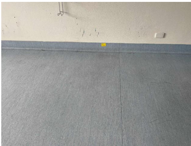
Line ID 28: Internal, Geriatric Unit Ground Level, Throughout, Floor Covering Throughout Rooms, Blue Vinyl Sheet - No Asbestos Detected
