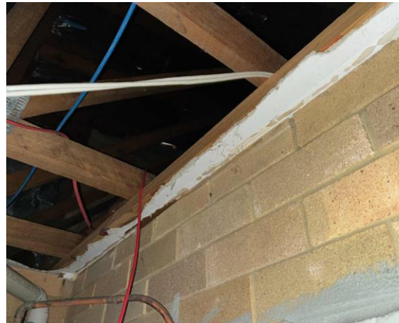
Line ID 33: Internal, Paediatric Unit, Adjacent NUM Room 30083, False Ceiling, Fibre Cement Sheet - Chrysotile Asbestos Detected
