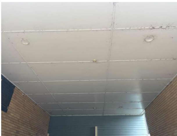
Line ID 16: External, Paediatric Unit, Throughout, Old Ambulance Carport, Ceiling, Fibre Cement Sheet - Chrysotile Asbestos Detected
