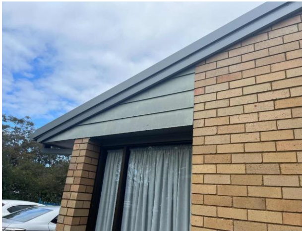
Line ID 14: External, Paediatric Unit, Throughout, Cladding around Windows and Awnings, Fibre Cement Sheet - No Asbestos Detected
