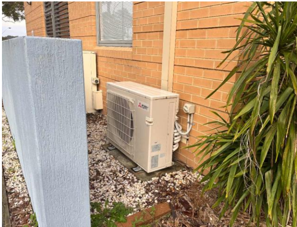
Line ID 87.1: External, Cancer Care Unit Ground Level, East Side, Mitsubishi AC Unit, R410A Hydrofluorocarbon (HFC) - Non ODS Refrigerant
