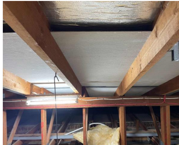
Line ID 23: Internal, Geriatric Unit, Rooftop Plant Rooms, Various Locations Throughout, Fibre Cement Sheet - No Asbestos Detected
