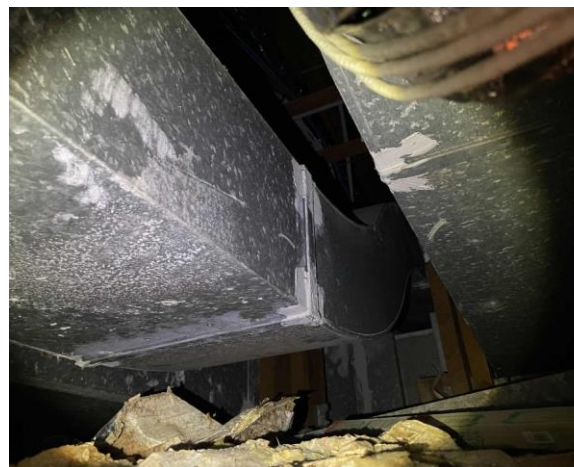
Line ID 37: Internal, Paediatric Unit, Ceiling Space, Ductwork Throughout, Mastic - No Asbestos Detected
