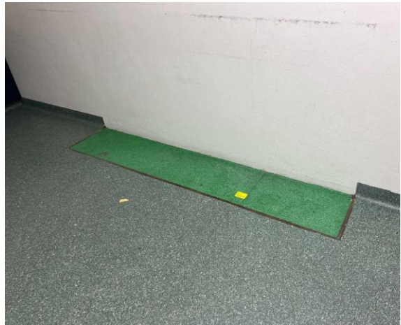
Line ID 46: Internal, Paediatric Unit, Southern Room 30089, Floor Covering, Light Green Vinyl Sheet and Paper Backing - Chrysotile Asbestos Detected
