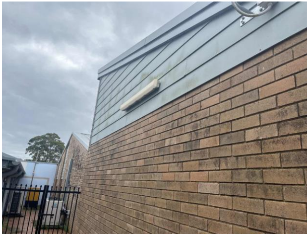
Line ID 86: External, Paediatric Unit, Throughout, Light Fittings, Ballast(s) and Capacitor(s) - Suspected PCB
