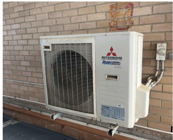
Line ID 89.1: External, Geriatric Unit Roof, Rooftop Plantroom, Mitsubishi AC units, R410A Hydrofluorocarbon (HFC) - Non ODS Refrigerant
