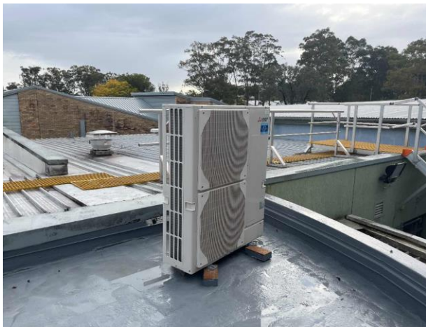
Line ID 89: External, Geriatric Unit Roof, Rooftop Plantroom, Mitsubishi AC units, R410A Hydrofluorocarbon (HFC) - Non ODS Refrigerant
