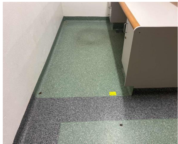
Line ID 44: Internal, Paediatric Unit, Short Stay Room 30069, Floor, Paper Backing under Green Vinyl - Chrysotile Asbestos Detected
