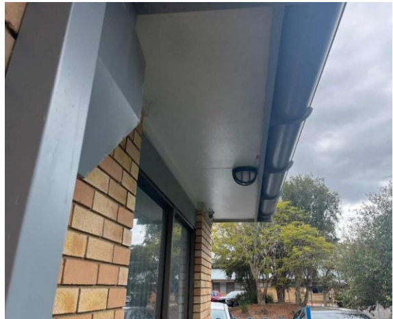
Line ID 15: External, Paediatric Unit, Throughout, Eaves, Fibre Cement Sheet - Chrysotile Asbestos Detected
