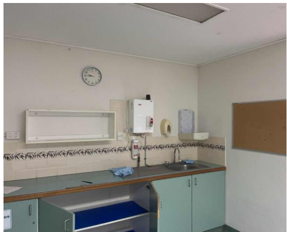
Line ID 85: Internal, Paediatric Unit, Kitchen 30074, Hot Water Heater, Above Sink, Internal Insulation - Suspected SMF
