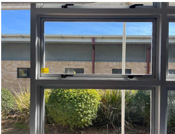
Line ID 30: Internal, Geriatric Unit Ground Level, Western Side, Window Frames, Mastic Sealant - No Asbestos Detected
