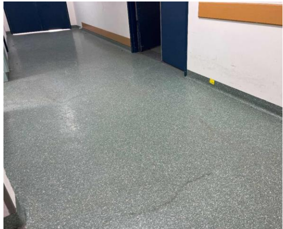
Line ID 48: Internal, Paediatric Unit, Throughout, Floor Covering, Green Vinyl Sheet - No Asbestos Detected
