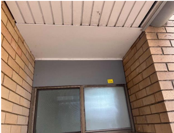
Line ID 12: External, Paediatric Unit, South Side, Infill Panel Above Window, Fibre Cement Sheet - No Asbestos Detected
