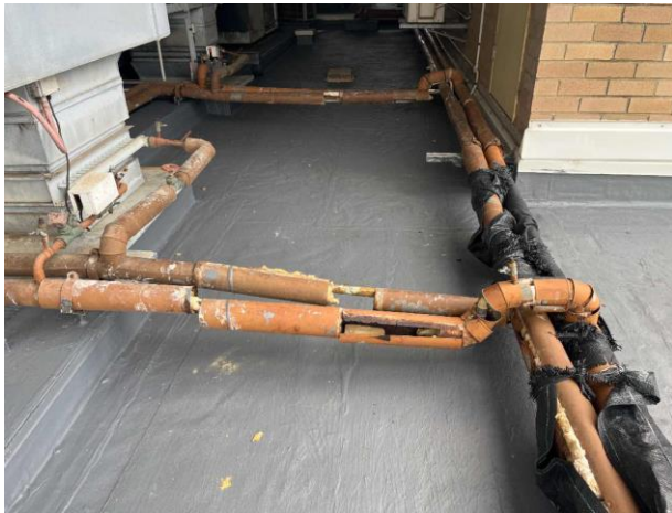
Line ID 61: External, Geriatric Unit Roof, Rooftop Plantroom, Pipework Throughout, Internal Insulation - Suspected SMF
