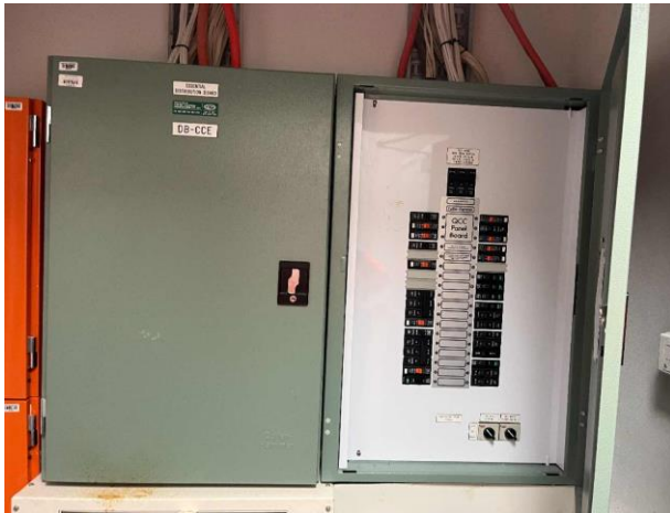
Line ID 20: Internal, Cancer Care Unit, Electrical Distribution Cupboard, Switchboard, HRC Fuses - Suspected Asbestos
