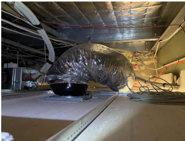
Line ID 76: Internal, Geriatric Unit Ground Level, Ceiling Space, Flexible Ductwork Throughout, Insulation Material - Suspected SMF
