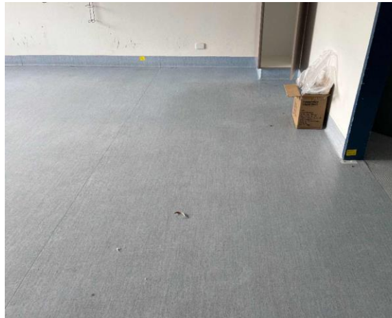
Line ID 27: Internal, Geriatric Unit Ground Level, Throughout, Below Light Blue Vinyl Sheet, Screed - No Asbestos Detected
