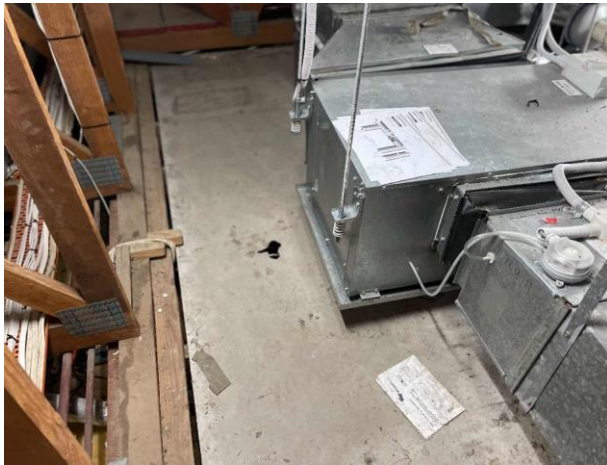
Line ID 22: Internal, Geriatric Unit, Rooftop Plant Rooms, Central Plant Areas on Southern Side, Compressed Cement Sheet - No Asbestos Detected
