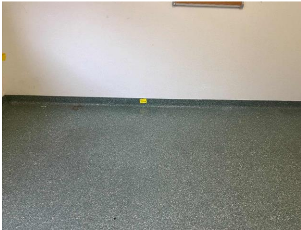
Line ID 45: Internal, Paediatric Unit, South Western Room 30094, Below Green Vinyl, Light Green Vinyl Sheet and Paper Backing - Chrysotile Asbestos Detected
