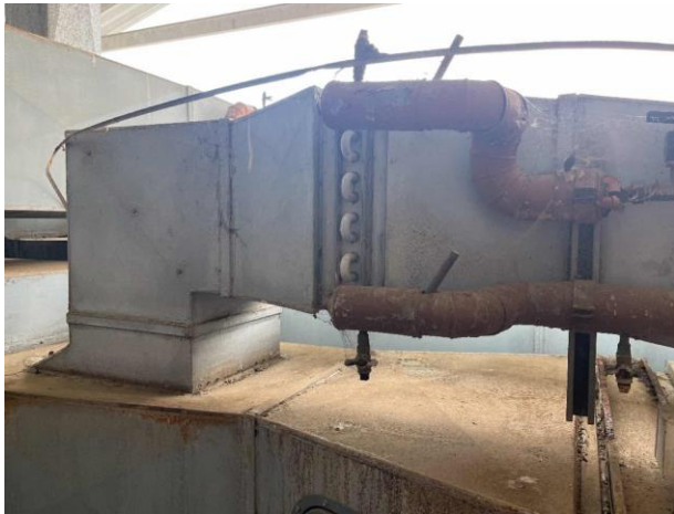
Line ID 8: External, Geriatric Unit Roof, Rooftop Plantroom, Within Western Ductwork, Millboard Insulation to Heating Coils - Suspected Asbestos
