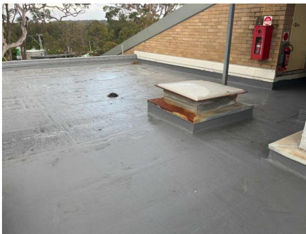
Line ID 5: External, Geriatric Unit Roof, Rooftop Plantroom, Floor, Bituminous Membrane - No Asbestos Detected
