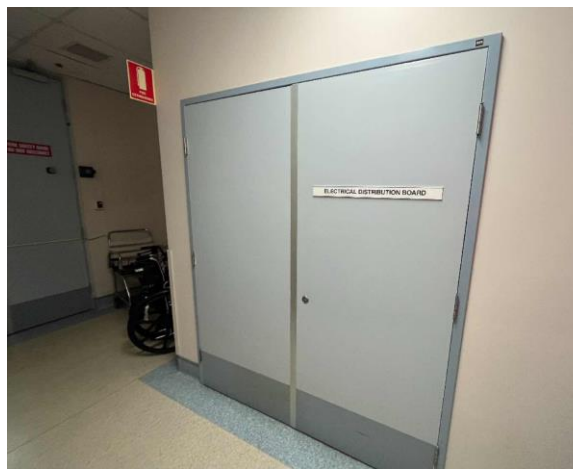
Line ID 19: Internal, Cancer Care Unit, Electrical Distribution Cupboard, Fire Doors, Fire Door Core - Suspected Asbestos
