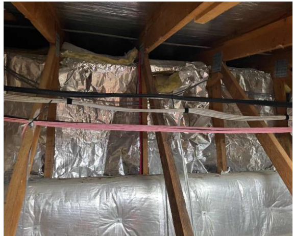
Line ID 75: Internal, Geriatric Unit, Rooftop Plant Rooms, Walls Throughout, Sarking Insulation - Suspected SMF
