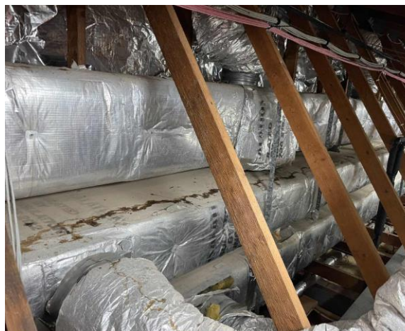
Line ID 73: Internal, Geriatric Unit, Rooftop Plant Rooms, Rigid Ductwork Throughout, External Insulation - Suspected SMF
