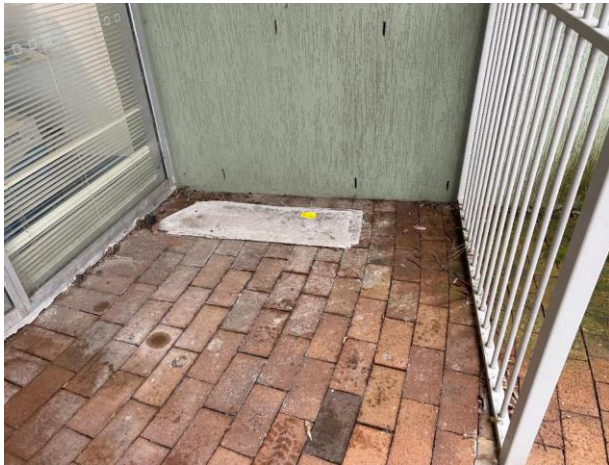
Line ID 1: External, Geriatric Unit Ground Level, South Eastern Side, on Floor, Adjacent Stairs to Roof, Fibre Cement Sheet Debris - No Asbestos Detected
