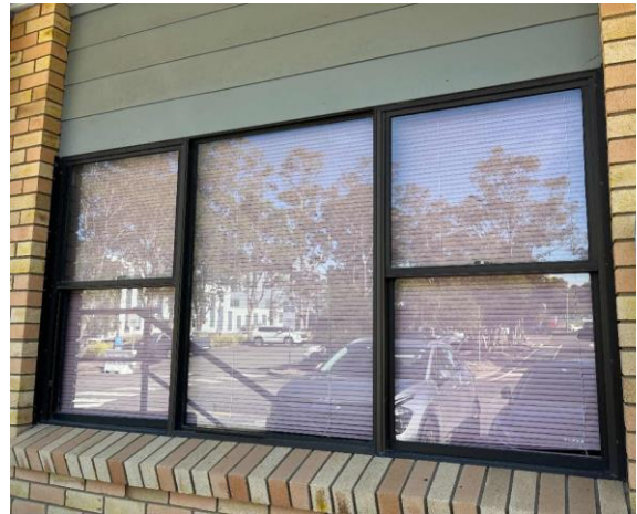
Line ID 9: External, Paediatric Unit, Throughout, Window Frames, Mastic Sealant - Chrysotile Asbestos Detected
