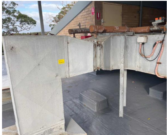
Line ID 4: External, Geriatric Unit Roof, Rooftop Plantroom, Ductwork Throughout, Mastic Sealant - No Asbestos Detected
