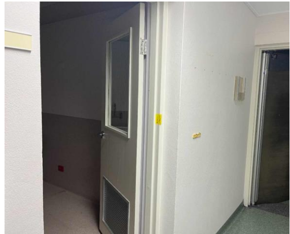
Line ID 54: Internal, Paediatric Unit, Throughout, Doors and Frames, White Paint - Lead Detected (0.005% w/w)
