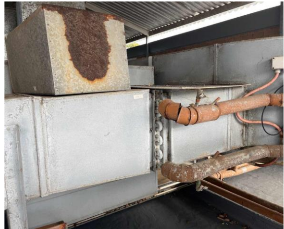
Line ID 7.1: External, Geriatric Unit Roof, Rooftop Plantroom, Within Eastern Ductwork, Millboard Insulation to Heating Coils - Suspected Asbestos
