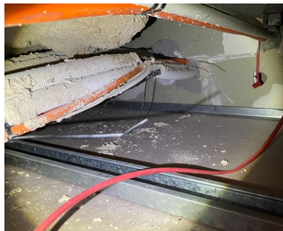
Line ID 25: Internal, Geriatric Unit Ground Level, Ceiling Space Above Doors to Cancer Unit, to Structural Beams, Vermiculite - No Asbestos Detected
