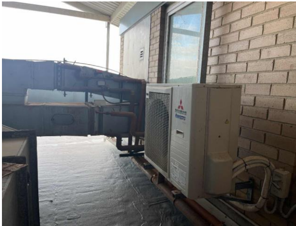
Line ID 89.2: External, Geriatric Unit Roof, Rooftop Plantroom, Mitsubishi AC units, R410A Hydrofluorocarbon (HFC) - Non ODS Refrigerant
