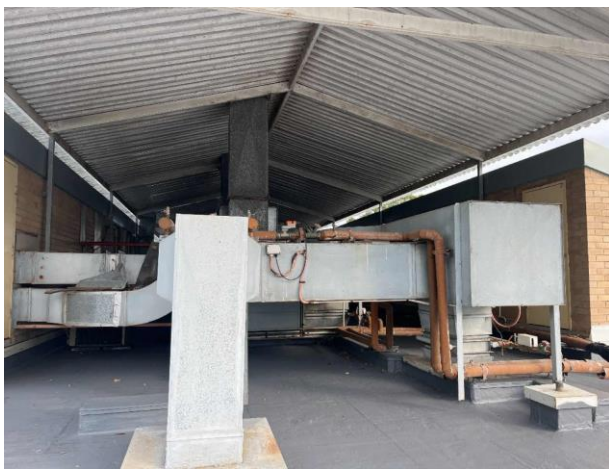
Line ID 51: External, Geriatric Unit Roof, Rooftop Plantroom, Air Conditioning Ductwork Throughout, Grey (Light) Paint - Lead Detected (0.02% w/w)
