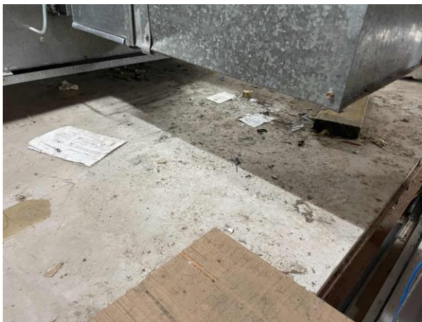
Line ID 57: Internal, Geriatric Unit, Rooftop Plant Rooms, South Side Throughout, Dust - Lead Detected (160 mg/kg)
