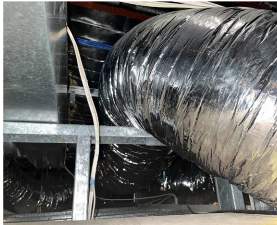
Line ID 65: Internal, Cancer Care Unit, East and West Sides, Flexible Ductwork, Internal Insulation - Suspected SMF
