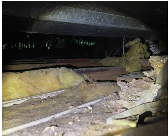
Line ID 83: Internal, Paediatric Unit, Ceiling Space, Throughout, Insulation Batts - Suspected SMF
