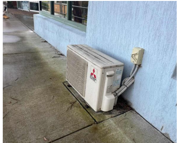
Line ID 88: External, Cancer Care Unit Ground Level, South Side, Mitsubishi AC Unit, R410A Hydrofluorocarbon (HFC) - Non ODS Refrigerant
