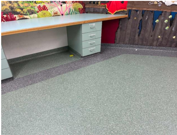
Line ID 41: Internal, Paediatric Unit, Procedure Room 30073, Below Green Vinyl Sheet, Paper Backing - Chrysotile Asbestos Detected
