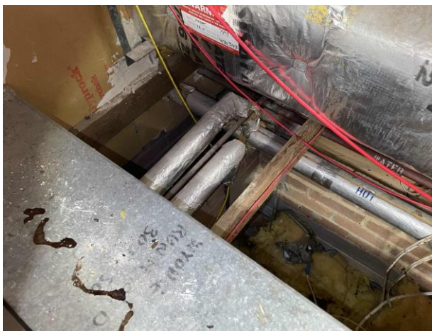
Line ID 72: Internal, Geriatric Unit, Rooftop Plant Rooms, Pipework Throughout, External Insulation - Suspected SMF
